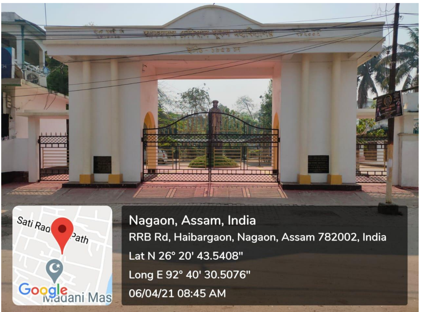
Fig: Main gate entry point of college
